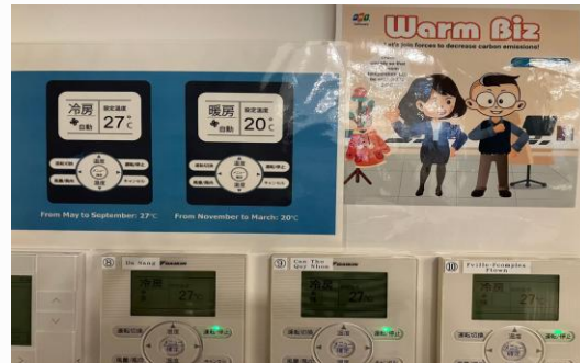
Promoting CoolBiz, WarmBiz: setting office temperature at 27°C from May to September, at 20°C from November to March
